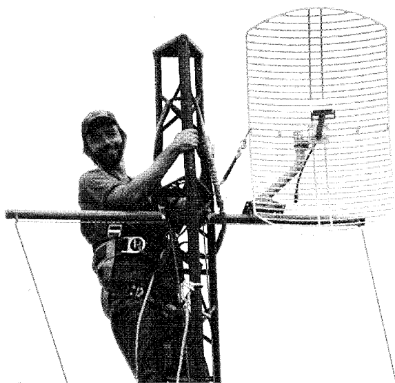
Figure 7-3—Height is important for any HSMM installation. In this photo, Daryl, KG4PRR, is installing an HSMM parabolic dish antenna at the home of K4RBZ.
