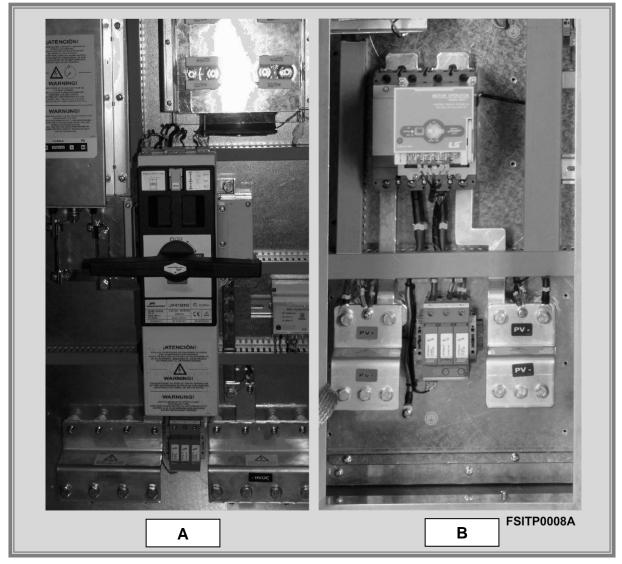
Figure 2.8 View of DC connection area with on-load disconnector (A) and circuit breaker (B)
