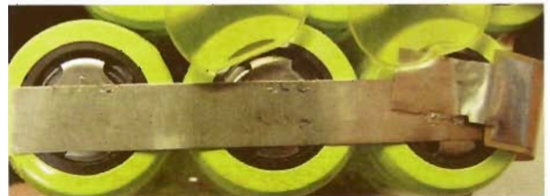
These insufficient welds aren't fully on their respective tabs, indicating poor quality processes. Bad welds are the most common problem in aftermarket battery packs, followed by blown welds.
