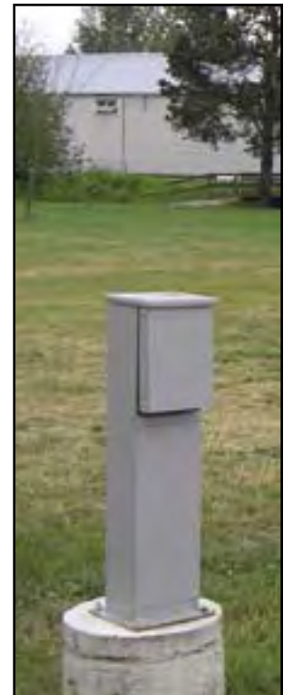
Battery Recharge Outlet – Maple Ridge Fairgrounds, Maple Ridge, B.C. photo credit: Donna Rodman
