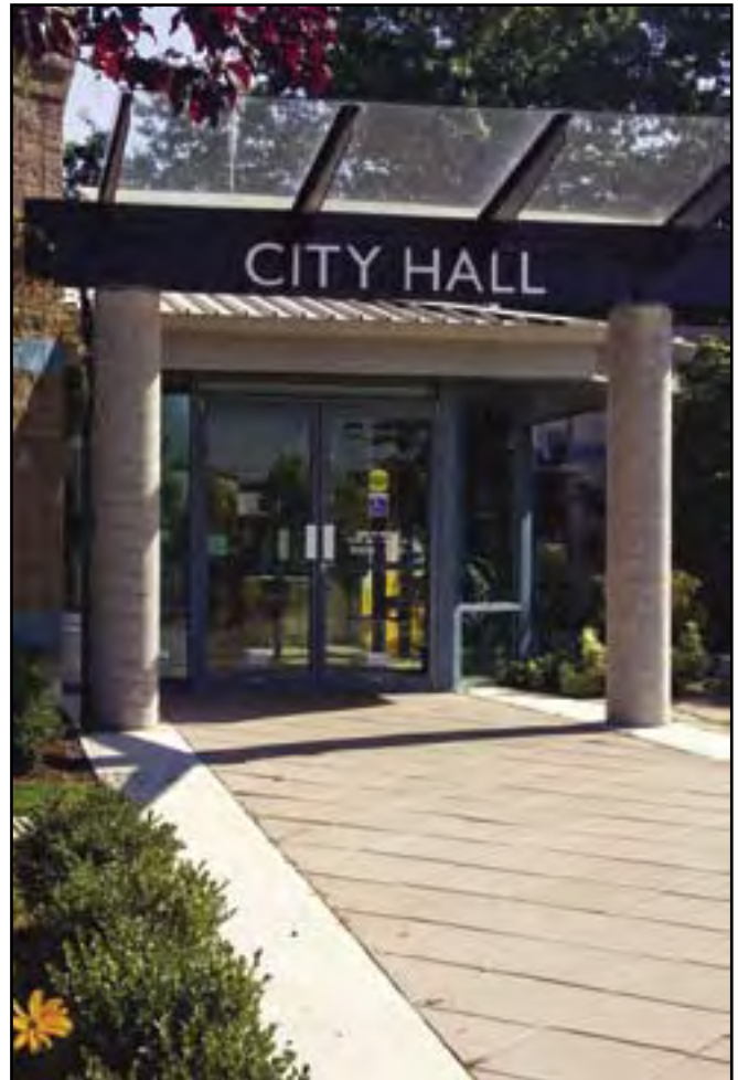
Accessible Building Entrance, Pitt Meadows City Hall, Pitt Meadows, B.C. / photo credit: Manfred Wuensche
