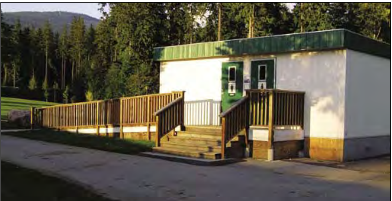
Outdoor Public Washroom – North Vancouver, B.C. / photo credit: Donna Rodman
