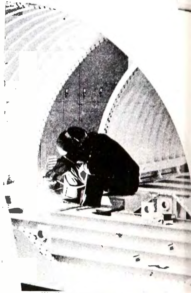
Westinghouse Electric Corporation Modular Portable Survival Shelter Under Construction
