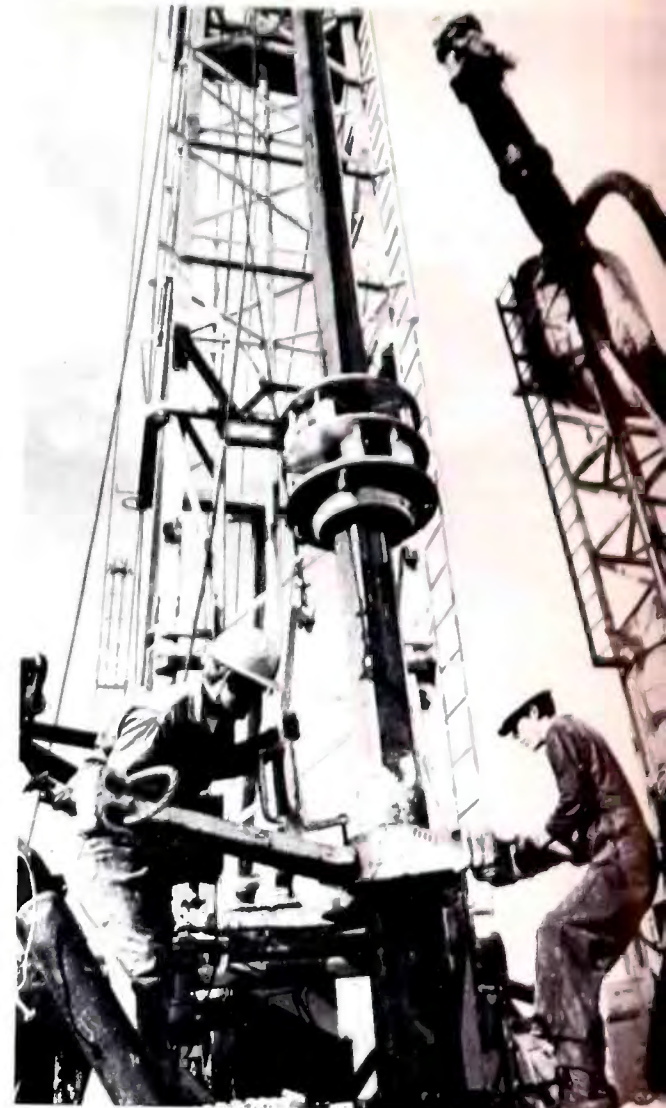
Westinghouse Electric Corporation Drilling Rigs for Rescue
