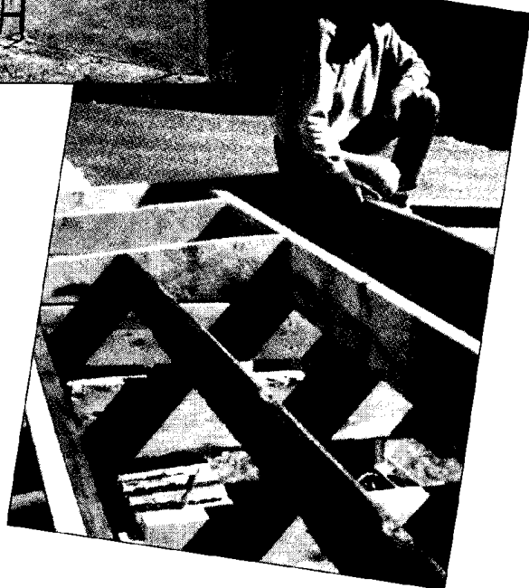
Catherine Wanek of Kingston, New Mexico, opted for a post-and-beam skeleton for her two-story greenhouse. She felt it would offer more stability.
