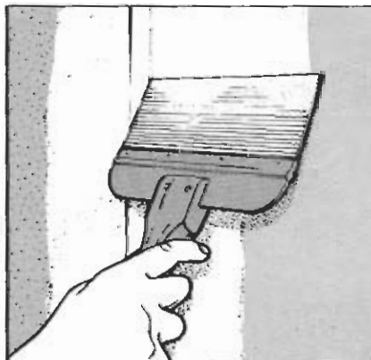
19 Once both sides of the tape are embedded in the joint, add another coat of compound to one side using an 8-in. knife.
