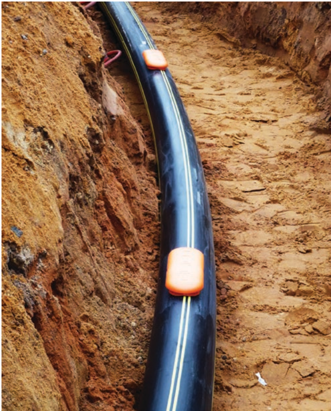
Fig.39: ELIOT Innovative solutions RFID tags on plastic (HDPE) gas pipe.
