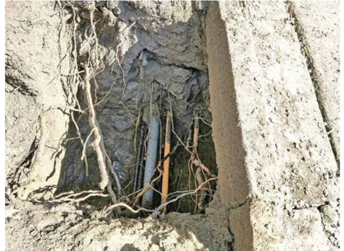
Fig.36: a ‘potholed’ site showing tree roots and utility cables. Potholing can be done to either locate services with certainty, or to make repairs once a leak or break has been located. Image source: Core Engineering, Inc.
