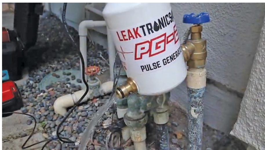
Fig.20: the Leaktronics PG-2 pulse wave generator connected to a domestic water pipe.
