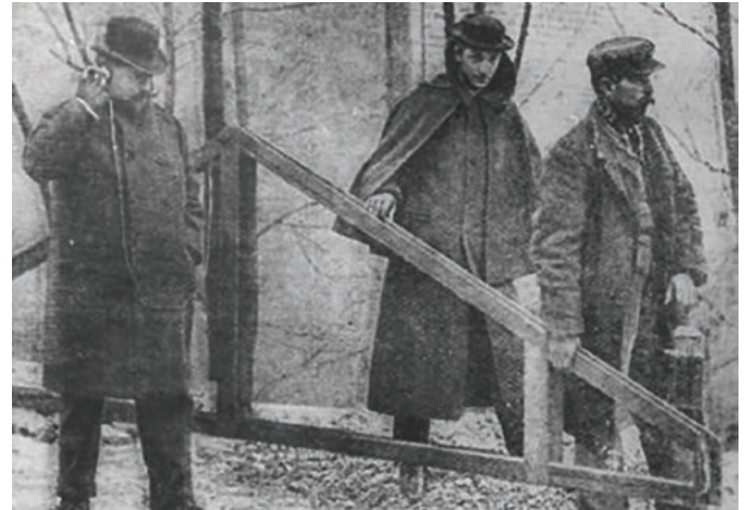
Fig.1: finding a buried cable using electromagnetic induction in Germany around 1910. The search coil is wrapped around a roof truss. A very large coil was needed, as there was no convenient means of signal amplification at the time.
