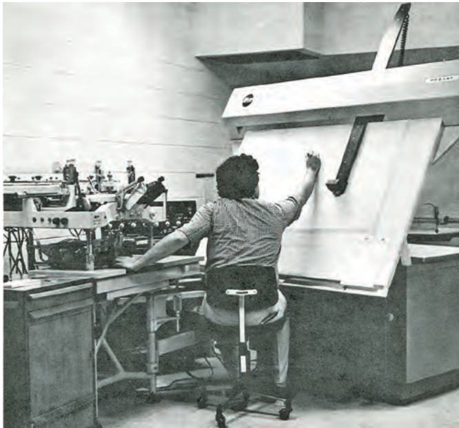
Fig.5: a photo from the "The Ontario Land Surveyor" of Winter 1979, showing the Kern PG2 stereo plotter connected to a Kern DC2-B Digitiser-Graphics Computer and an "automatic drafting table". Aspects of feature extraction from stereo photos were automated or semi-automated.
