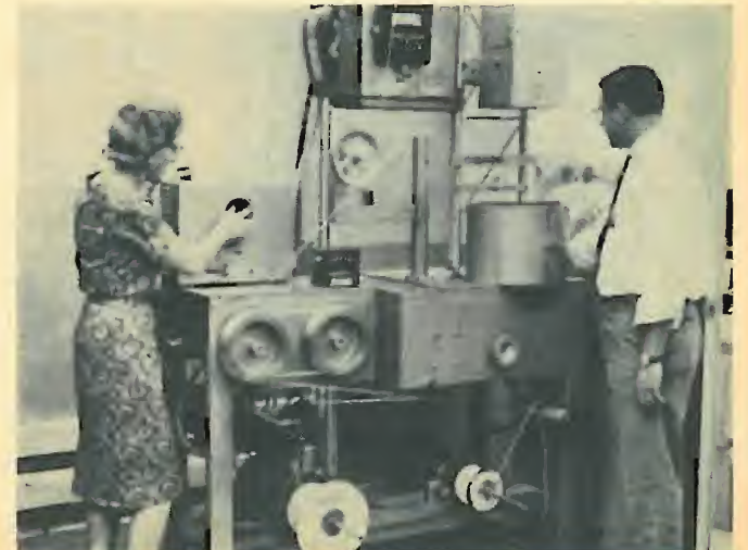
Fig. 3. The line drawing illustrates the previous method used by Lockheed Electronics Co. to dispense color-coded wire. In this case individual spools of color-coded wire were purchased from an outside vendor. In new method, shown in the photo, white wire is bought and up to three colors are applied by the in-plant machine to the exact lengths required for each job. This eliminated surplus and resulted in saving $43,500/yr.
