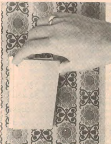
The metal touch plate simply clips into position over the grid plate.
