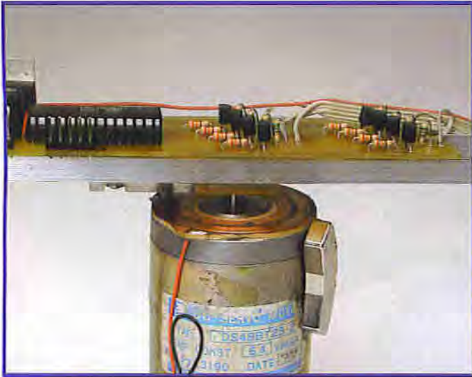
Figure 4. A slip ring provides the power supply to the rotational circuitry.
