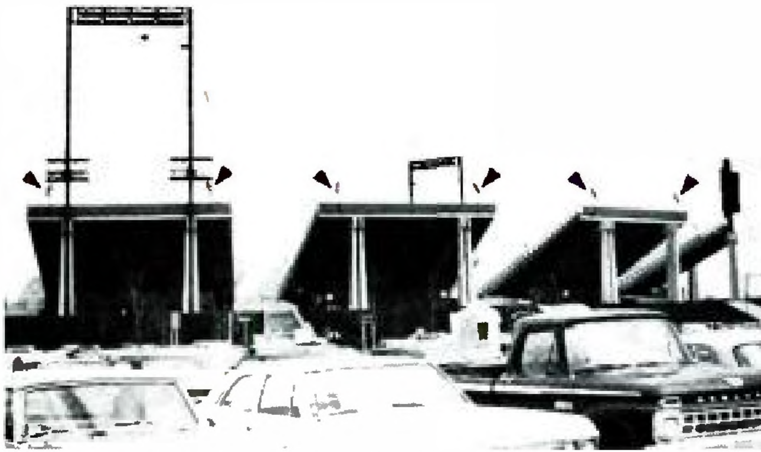
Fig. 1. Autostade Stadium — the arrows show the location of some of the 38 sound columns used for distribution.
