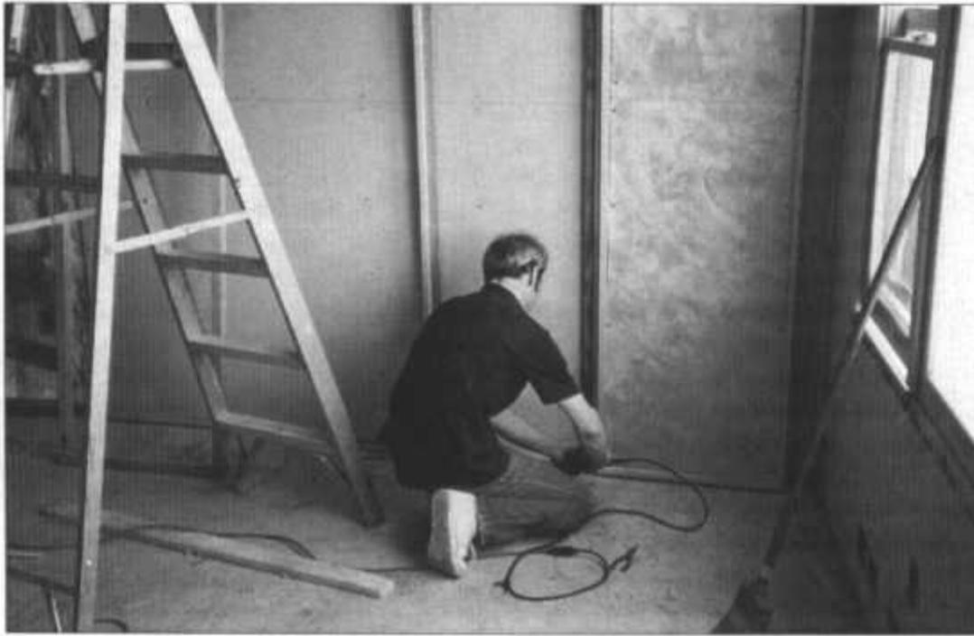
**FIG. 4: Master carpenter Rick Castillo attaches a bass trap to the wall with toggle bolts.**
