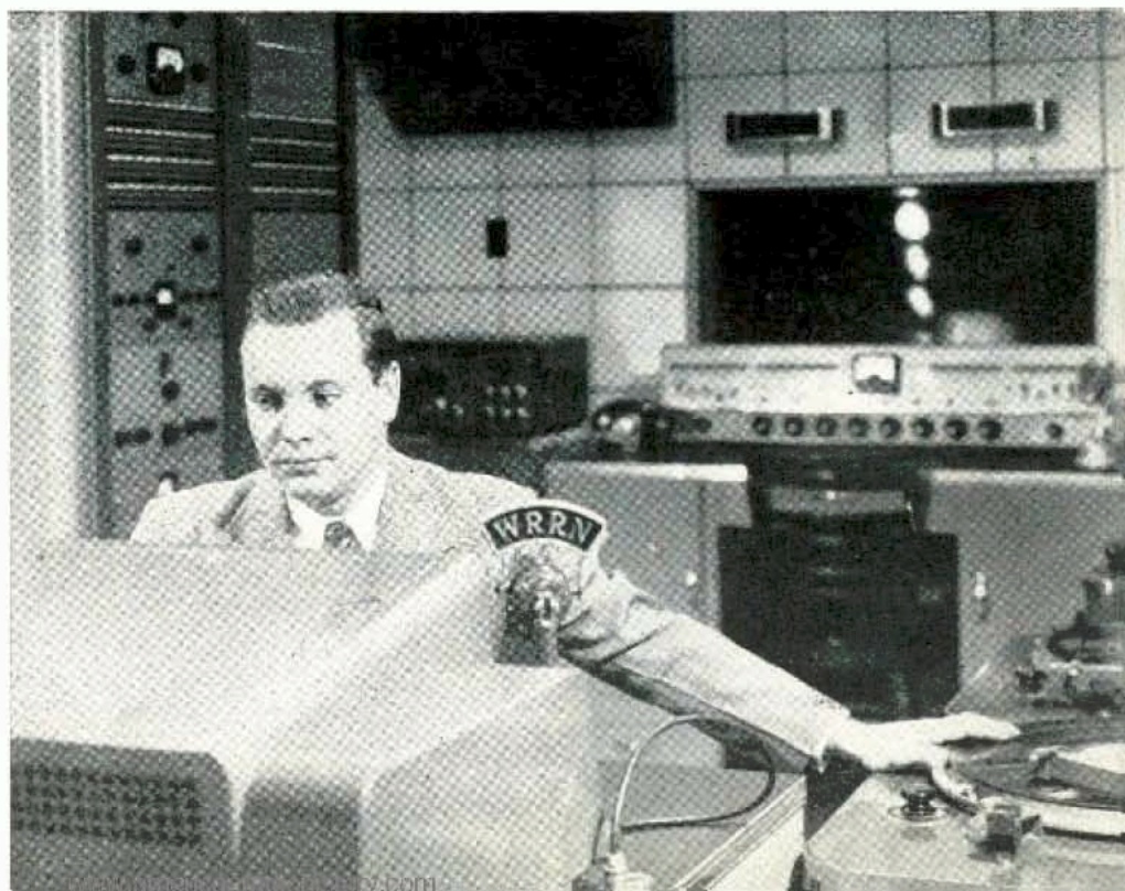
Fig. 1—The Master Control Room of WRRN, Warren, Ohio, showing the location of the control consoles, equipment racks, turntables and other facilities.
