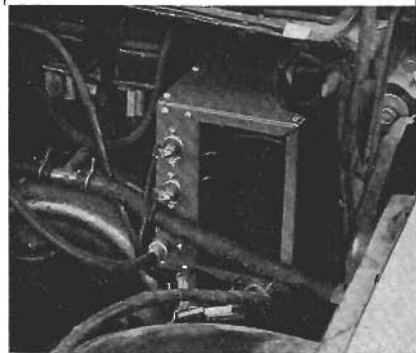
Fig. 5 (top) Regulator, terminals, and coaxial capacitor placements in shield box. (Bottom) Regulator shield box showing standard coaxial cable connector at end of generator field cable.
