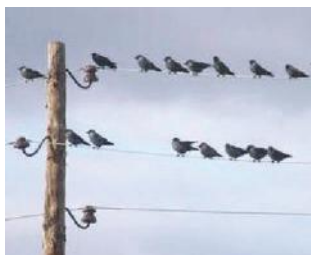
FIGURE 2.21 Birds don't get electrocuted when they sit on a power line because they do not experience a voltage "drop."
