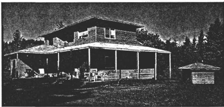
In this award-winning design, a fan pressurizes the crawl space, blocking radon entry. Heat is recovered from the exhaust air. The hut in the yard covers a tube that draws fresh air into the house.
